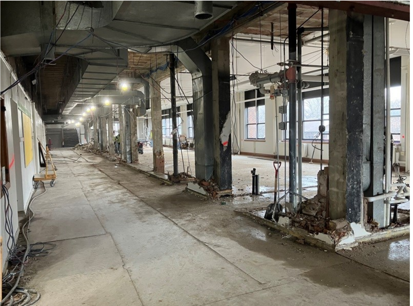
Third floor demolition (December 2023)
